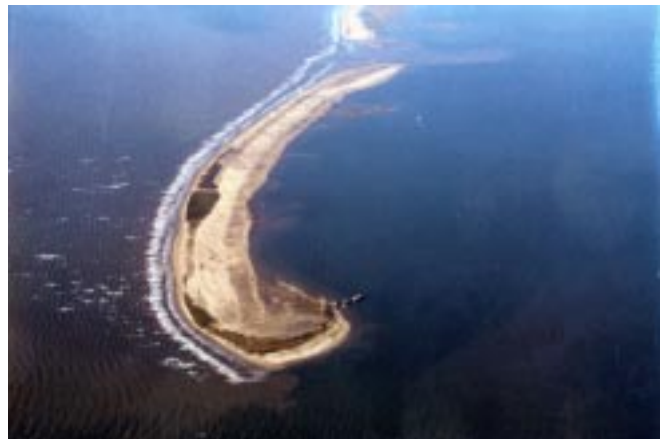
Dredged material was used to increase the height and width of East Island (TE-20) in 1999.
