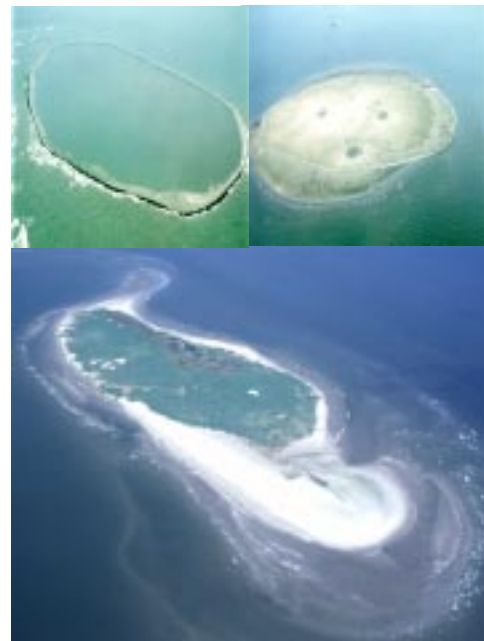
Wine Island Restoration project showing rock levee (top left) and dredge material (top right). Vegetation was later planted (bottom).
