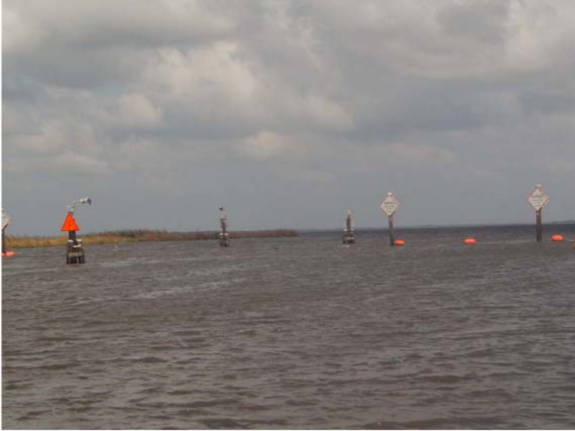
Photo #1 – Bayou Dupont Canal Weir. Approaching the Bayou Dupont weir from the Barataria Waterway, looking across the weir boat bay toward the Pen. Warning signs and navigation aids, or lack thereof, are shown on either side of channel through the boat bay. Note the damaged lights.
