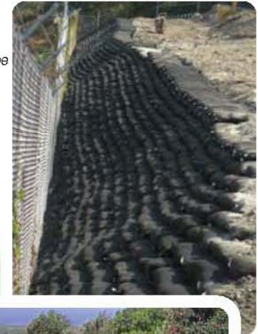
Deltalok® reinforced slope
