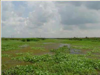
Pilot Canal After Backfilling
