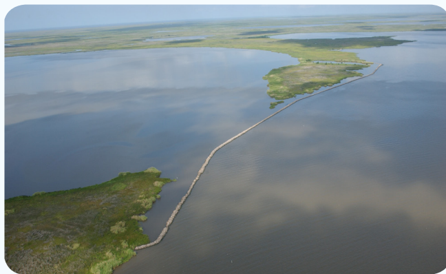
The Marsh Island Hydrologic Restoration project's features include shoreline protection, canal closures, and isolation of Lake Sand from Vermilion Bay with a rock dike on the northeastern edge of Marsh Island. View is looking west.
