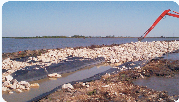
For the Brady Canal Hydrologic Restoration project, the narrow, eroding shoreline of Bayou DeCade was reinforced with rock in order to help restore the hydrology of the Brady Canal area.
