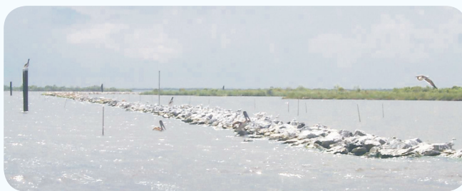
Part of the Gulf Intracoastal Waterway to Clovelly Hydrologic Restoration project, the constructed rock breakwater located in Bay L'Ours assists in reducing wave energies before they impact the shore.
