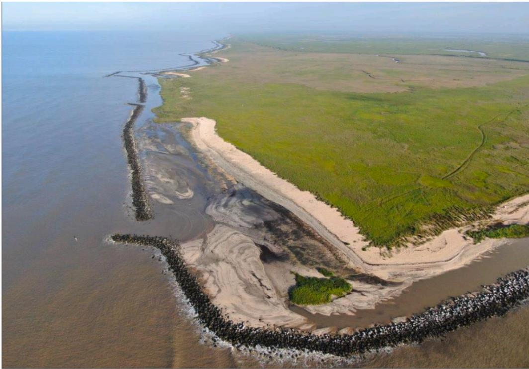
Fig. 17. Breakwater composed of lightweight aggregate, bedding stone, and large armor stone [97].
