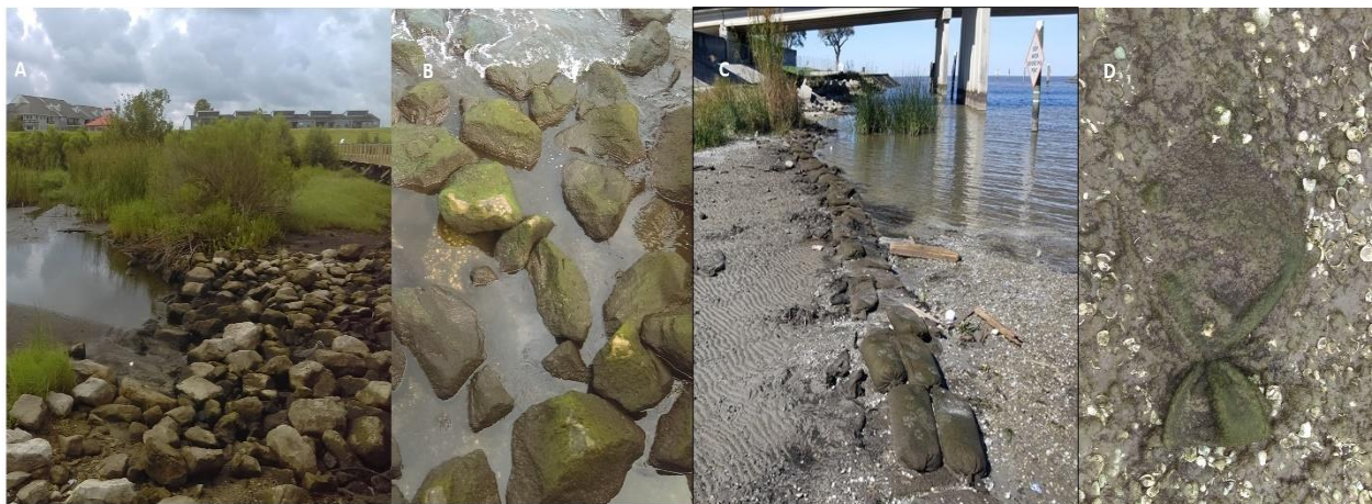
Figure 16 Comparison and close-ups of the retaining walls used at the Bucktown Marsh (~10' wide border of rock, A & B) and at Bayou St. John Urban Marsh (~2' wide border of sand filled bags, C & D)
