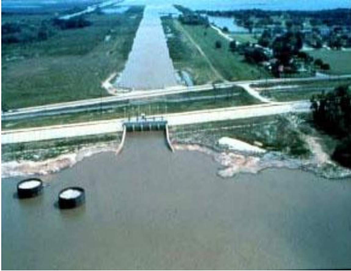
Figure 2.3-Aerial view of Caernarvon Diversion Structure (Day 2005).
