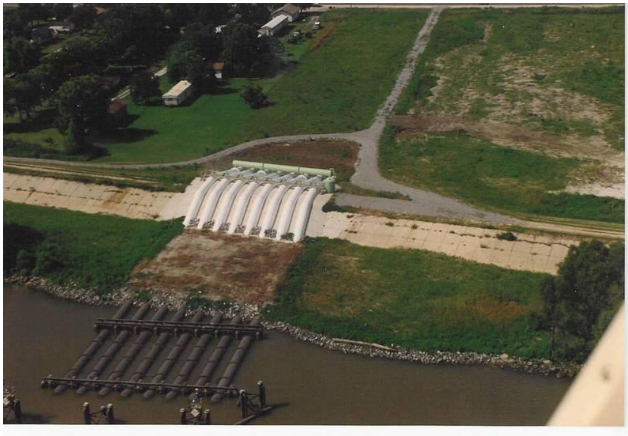
Figure 2.7-The West Point a la Hache Freshwater Diversion (LDNR)
