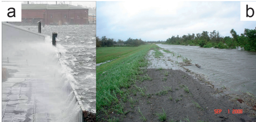
FIG. 2. Photographs during Gustav of (a) waves overtopping the IHNC walls near the Ninth Ward and (b) surge overtopping the earthen levee near Braithwaite. (Courtesy of Nancy Powell, USACE.)
