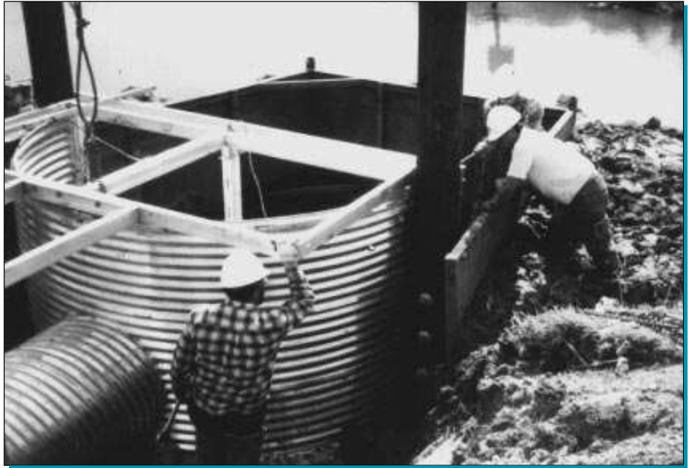
Workers install one of three double-barrel corrugated aluminum pipes at the East Mud Lake Project. Each pipe has a variable crest weir inlet section with a vertical slot.
