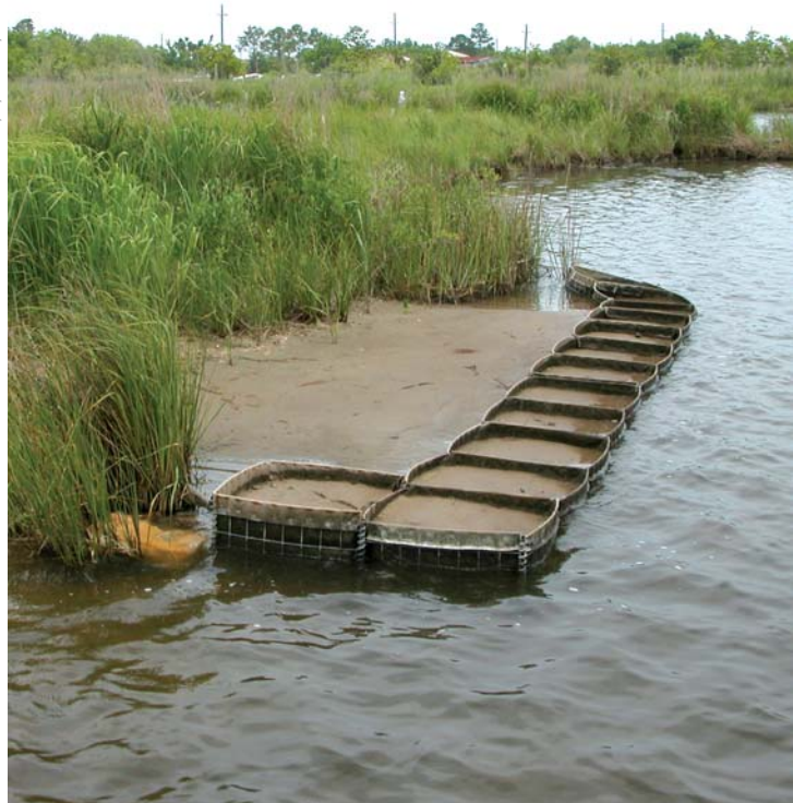
Some sites require artificial barriers to hold sediment in place until vegetation takes root. Here pop-up baskets of metal and fabric keep sediment from washing away.
